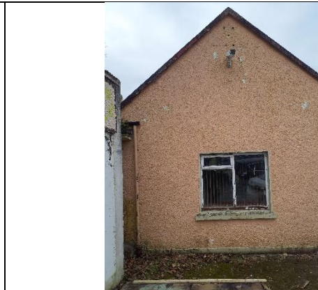
Plate 2: North side of old fire station
