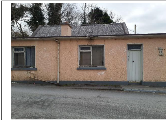
Plate 1: West side of old fire station
