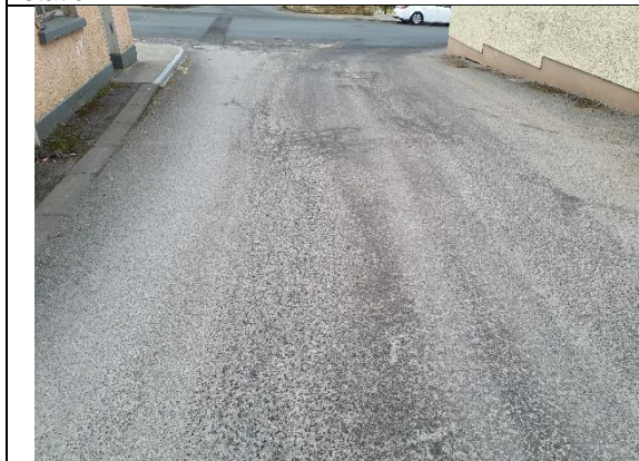
Plate 5: Road sloping south-westward on west side of site.
